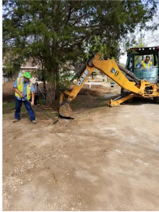
Culvert replacement at E. Walcott
